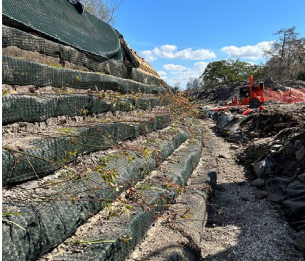
Stream Bank Stabilization and Planting Construction
